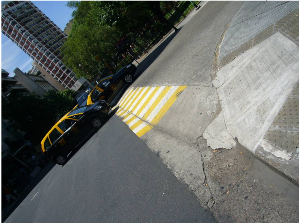
7-Detalle rampa-cuneta
